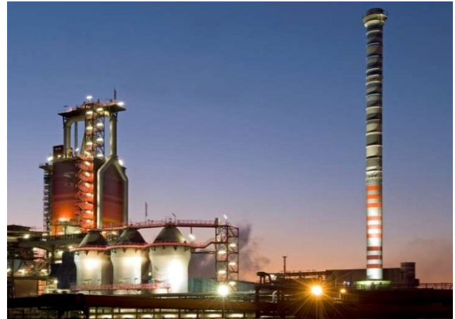
© thyssenkrupp Steel Europe
